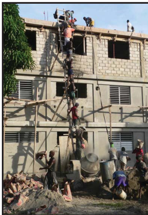
Workers build the 3rd story of the James Stine College with a concrete assembly line.
